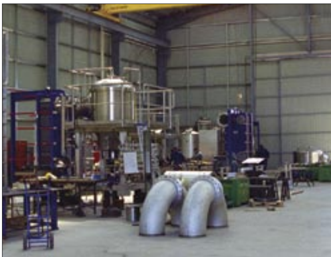
Centritherm assembly line in the new manufacturing facilities.
